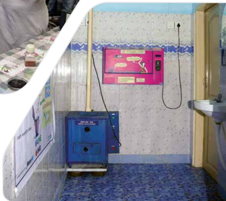
Sanitary napkin dispensing unit and the green disposing unit installed at the WASHE schools
